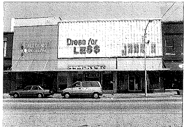
The signs on these buildings are completely inappropriate. Upper level window openings and detailing have been covered and the signs now totally dominate both buildings.
