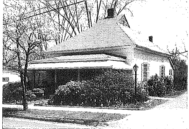
The gable-on-hip roof may be seen on several Granite Street houses in Hogansville. It is a very distinctive roof type and is an example of how important roof form can be in defining the character of a house.
