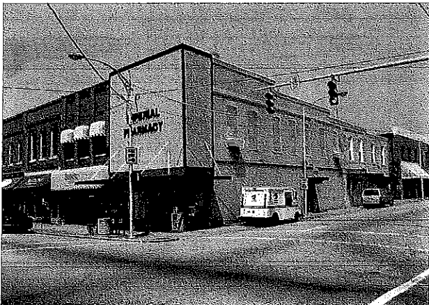
This brick building has received a variety of insensitive treatments. The original brick has been stuccoed over, metal siding has been applied to the front facade and second level openings have been boarded up. Obviously, this building detracts from the historic structures nearby.
