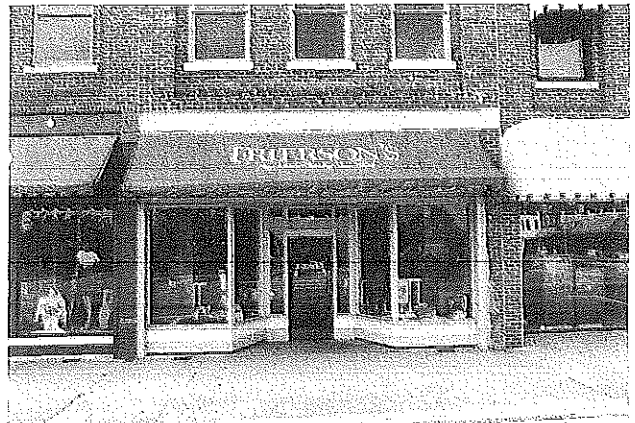
Looking much as it probably did originally, this storefront serves as an excellent example of sound commercial building preservation.
