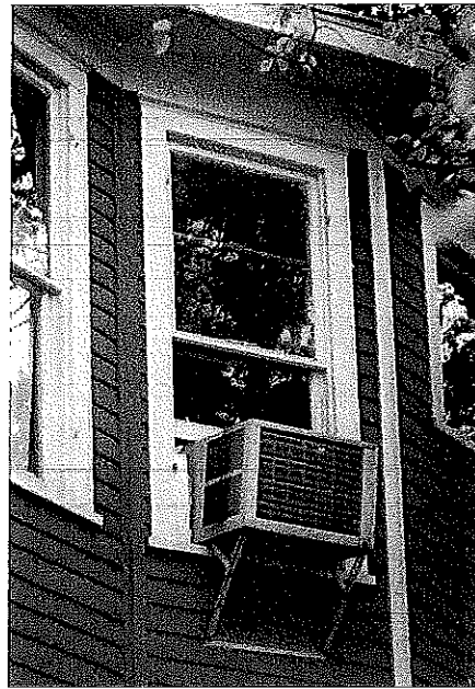
Window air conditioning units should never be positioned on the front facade of a house, but rather to the rear or at a view-obstructed location.
