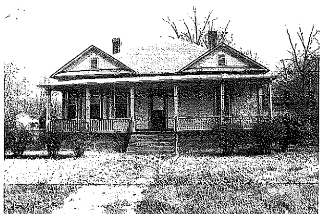
The gutters and downspouts on this house are barely noticeable; they are well-positioned and unobtrusive.
