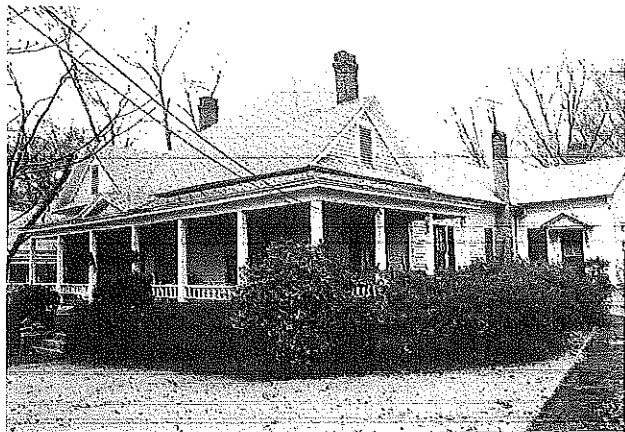
This house exhibits four properly-maintained brick chimneys that contribute to the building's architectural character.
