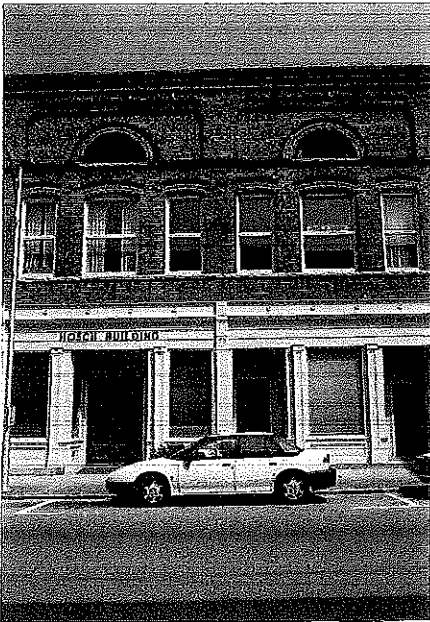
The upper level of this well-preserved building is in use as office space.
